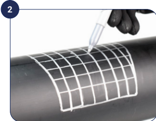
Mark the scraping zone
