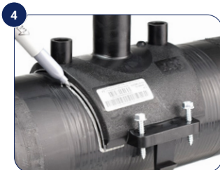
Mark the welding zone
