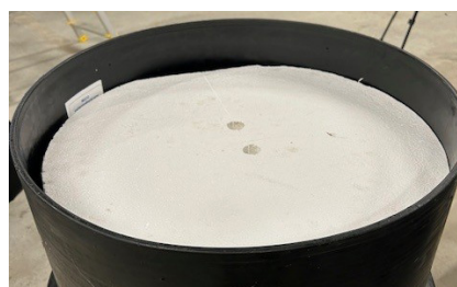
Isolering under locket
